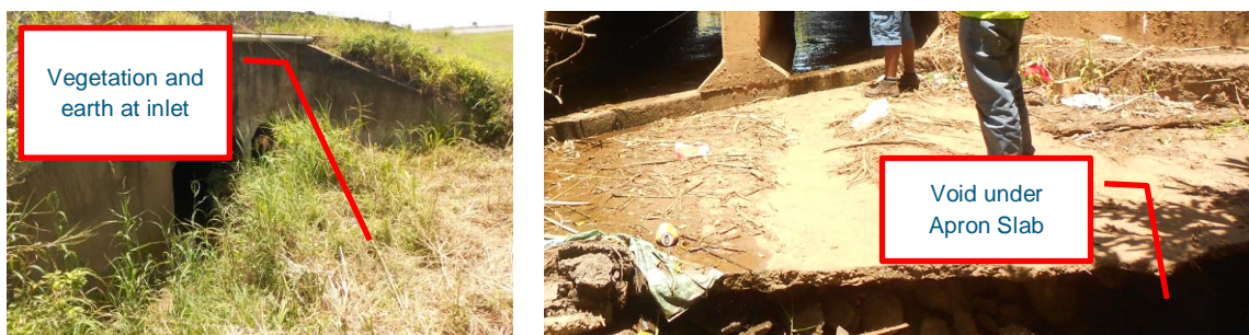
Figure 3-1: Inlet vegetation (left) and failed outlet apron slab (right)
