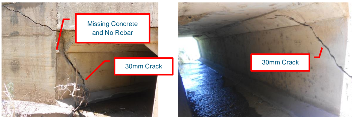
Figure 3-2: Cracks in the culvert barrel and wing walls
